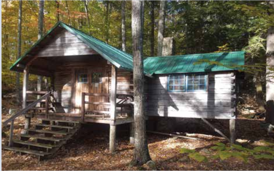
Cabin on Stonedam Island with new roof and support posts
